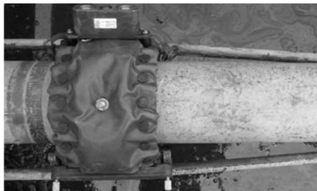
**Fig. 4.** An applied ring on a tube and two heating pipes that are bent out for application of the ring
