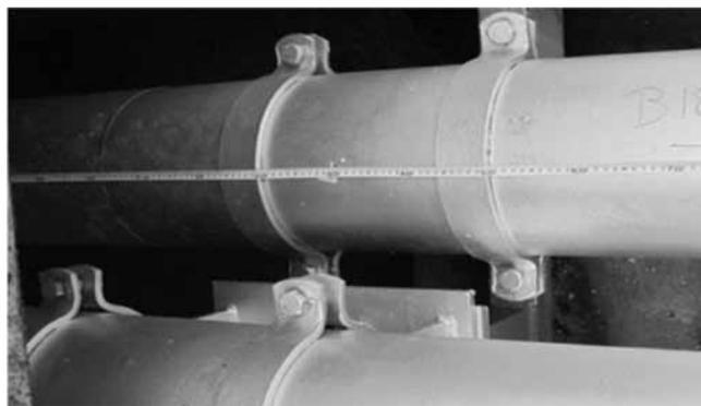
Fig. 5. Supportin clamps on the pipes
